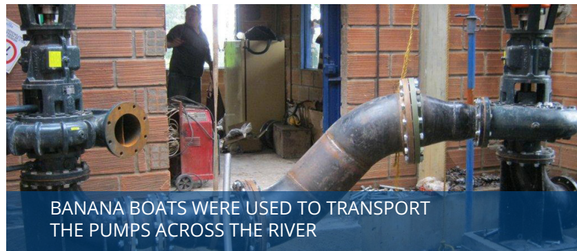
VERTICAL MOTORS TO AVOID DAMAGE FROM FLOODING
